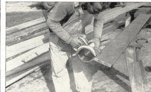
↑ Lumber is cut to length or ripped in a minimum of time to speed up all types of construction.
