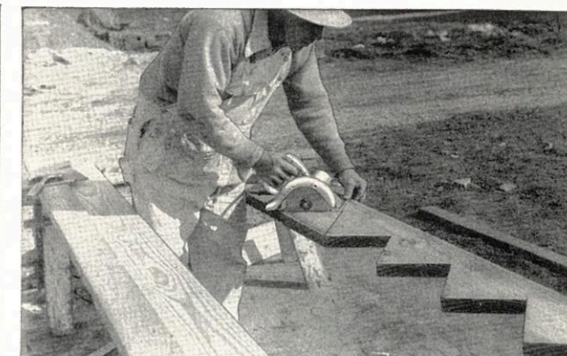
↑ The Home-Utility Saw cuts stair stringers in a fraction of the time required with a hand saw.
