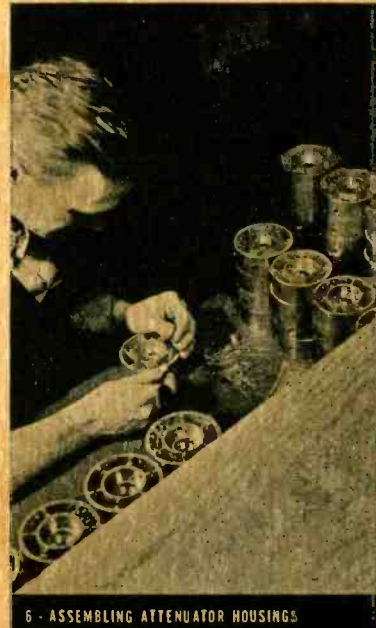
6 - ASSEMBLING ATTENUATOR HOUSINGS
