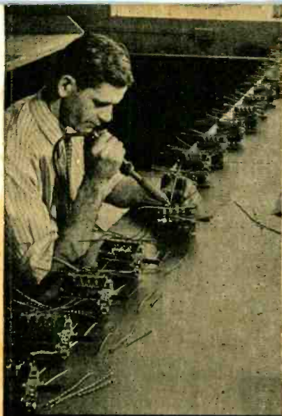
19 - WIRING FREQUENCY CHANGE SWITCHES
